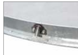
drainage stub pipes
