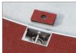
box installed in throwing facility surface
