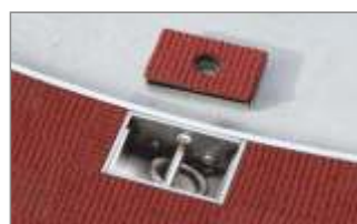
box installed in throwing facility surface
